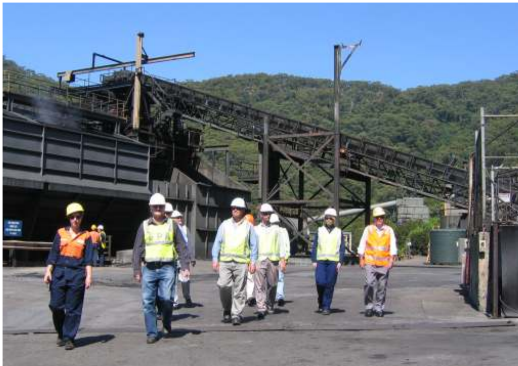
A delegation from the NSW Department of Environment, Climate Change & Water during a visit to Coalcliff Cokeworks
